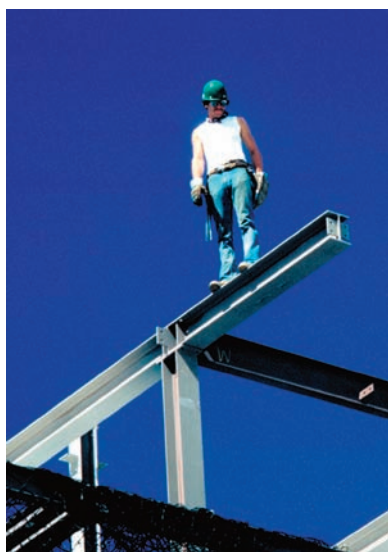
Fig. 12-3 A construction worker balanced on a steel beam is in static equilibrium but is more stable parallel to the beam than perpendicular to it. (Robert Brenner/PhotoEdit)
